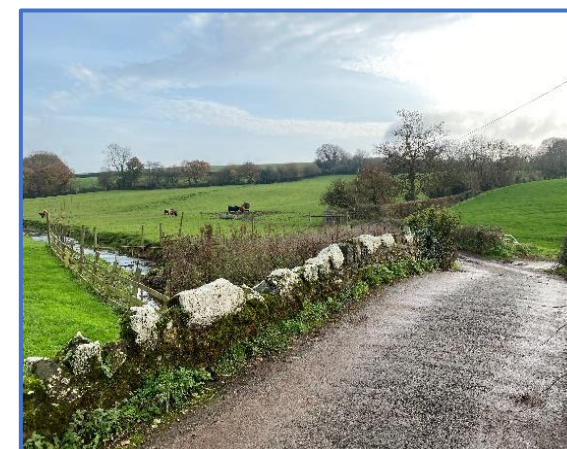
The bridge over the River Weaver at Garlandhayes Farm
